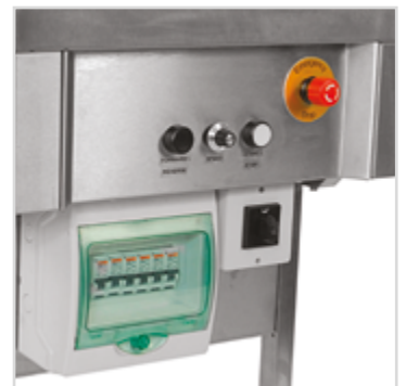
Control panel & splash proof distribution switch board
